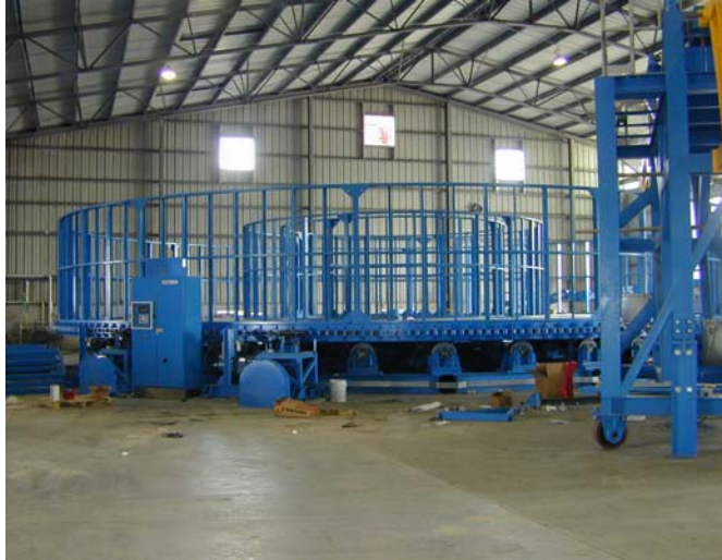
1000Te Umbilical Carousel Installation - Texas USA
